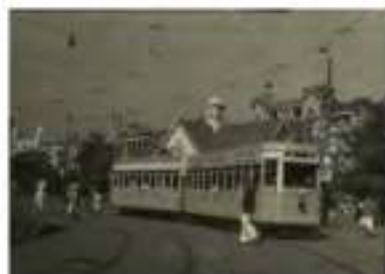
Introduction of public transport: Electric Tram
