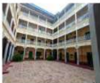
View of Courtyard
