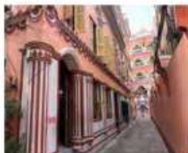
Entry to Ashram area (renovated)
