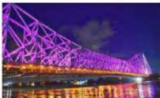
Night View of Howrah Bridge
