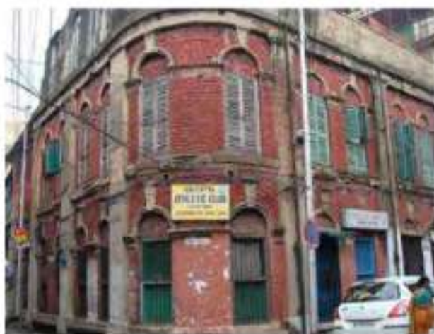
Residential Building: mid 20 th century, Plot No. 22B, Hemendra Saa Street (Dorjapara- North Kolkata), Ownership- Private, Status- Unprotected
