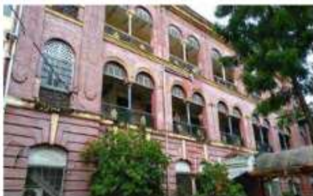
Arched veranda with CI ornamental Grill and rusticated exposed brick walls at ground floor
