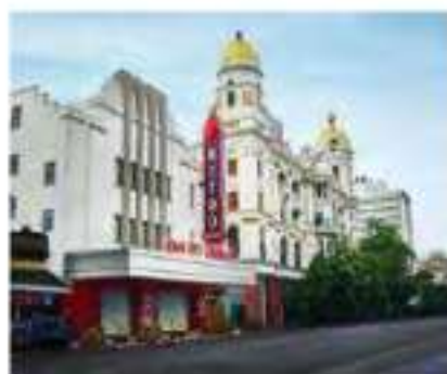
Métro Cinema after renovation in 2022
