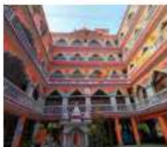
Guest House complex (new extension)
