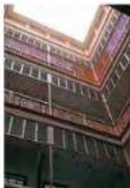
Interior view from courtyard
