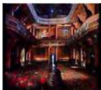
Interior view of the hall before restoration
