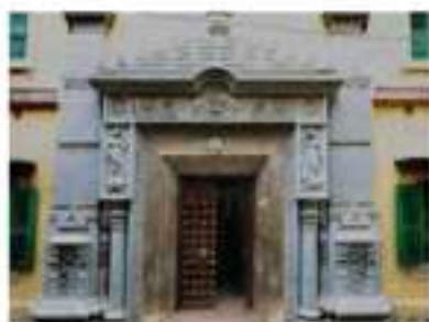
View of Entrance :
