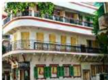
Rail Castle , post-Independence era, Usage- Residential Plot No. 12, Alamy Road, Chakraborty (South Kolkata) Ownership- Private, Status- Unprotected
