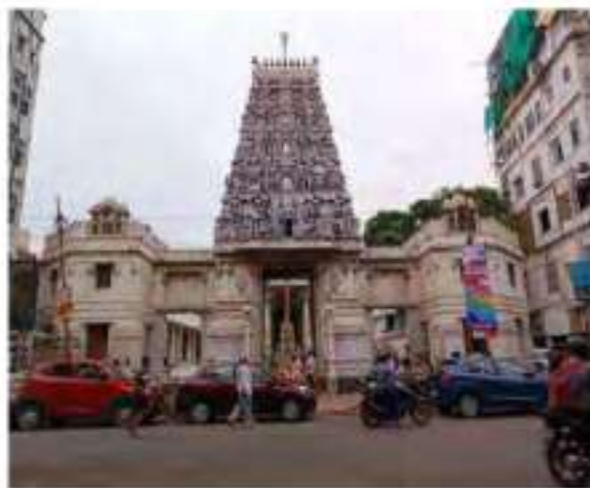
Exterior view of the 'Gopuram'
