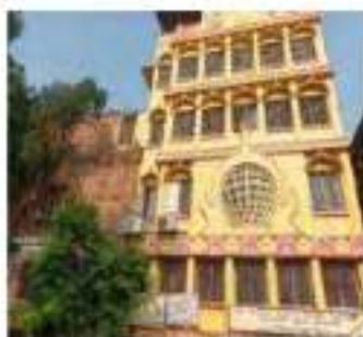
New Adjacent Block
