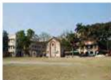
View of the School building from playground
