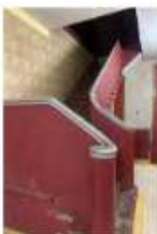
Stair to upper floor PC: Danghamsite.com
