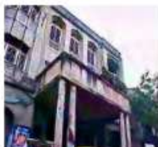
Minerva Theatre before restoration
