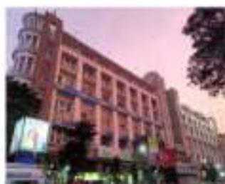
Hindustan Building (JTC), Protected - Art Deco
