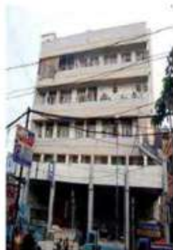
Gurnea House at present- facade totally razed
