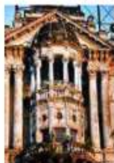
Central bay (Before Restoration)
