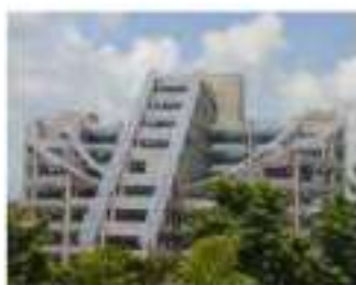
New India Assurance Bldg at Rajarhat- New Town
