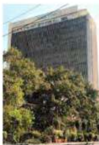
Side view of Tata Centre
