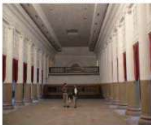
Figure 15 The Town Hall post restoration.
