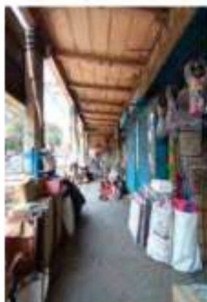
Below the grand facade veranda-squares section
