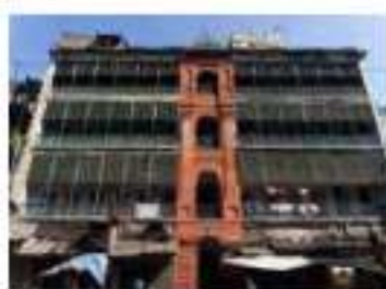
representative example of Residential Buildings, MG Road, Barabazar
