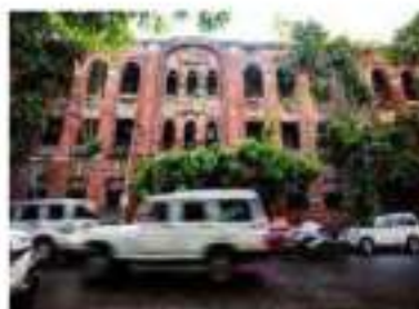
Front view- Left side- neglected
