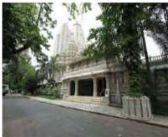
Side view- Siva Sanyas- the auditorium at basement
