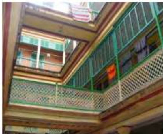
House of B. Sircar Johannes (1917-21), Usage- Residential Plot No.114 B, Howbazar Street, (Central Kolkata), Ownership- Private, Status- Unprotected With C.I. Grill and wooden fixed louvers (Jhill)- a typical feature
