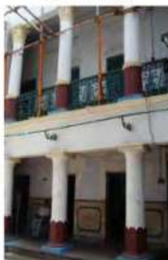
View from courtyard
