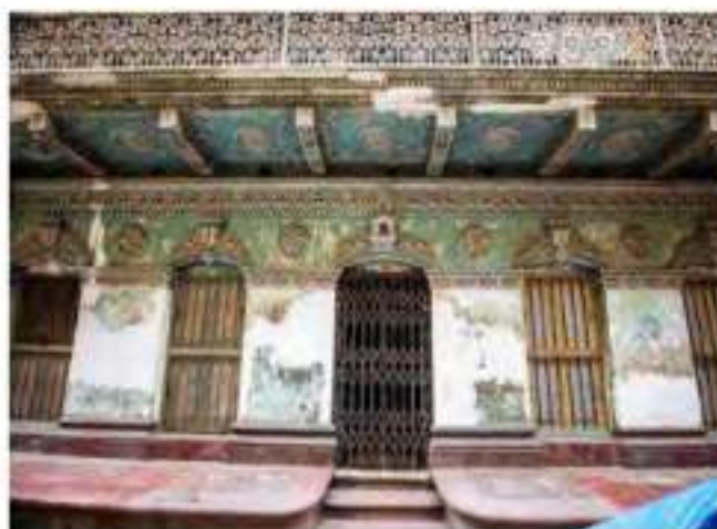
Elaborate ornamental stucco work on the interior face
