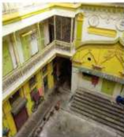
View from courtyard
