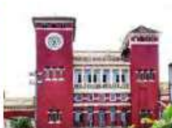
Howrah Station (at present)
