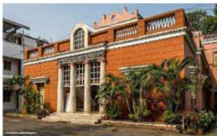
Figure 32 The Kolkata Police Museum. (Source: The Concrete Research)
