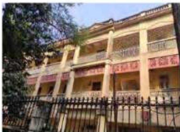
View of the Dharanishala from the internal courtyard
