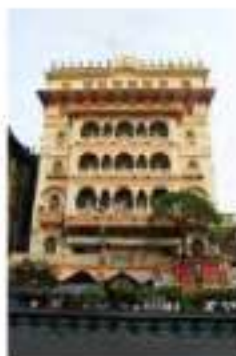
Ram Mandir - CR Avenue Status- Unpreserved
