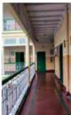
View of upper floor Terrace
