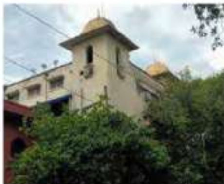
Cupola of corner - a landmark feature
