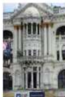
Central bay (after Restoration)
