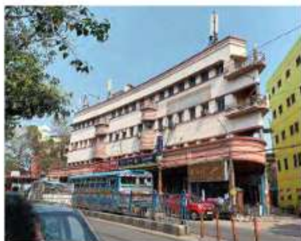
House of Dr. Nilratan Sircar, (Mid-20 th century), Usage- Residential (Past), Commercial (Present) 61, MG Road (Central Kolkata), Ownership- Trust Property, Status- Unprotected
