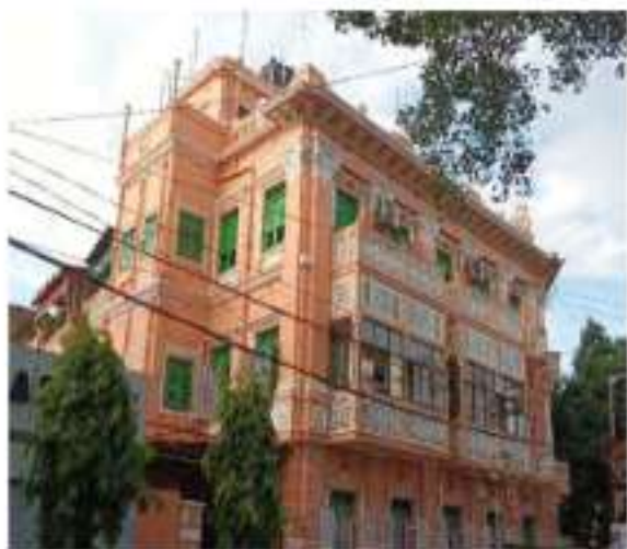
Residential House, Usage- Residential cum commercial Pin No.81A, J.L.Nehru Road (South Kolkata), Ownership- Private, Status- Unprotected
