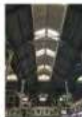
use of transparent sheet on roof for the natural light
