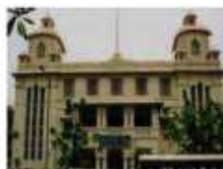
Mahajati Sadan- Pre. No. 188, CR Avenue Status- Preserved
