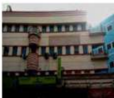
Semi-circular protruded veranda
