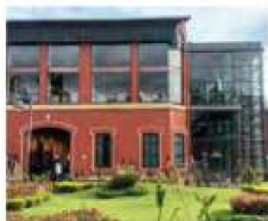
Rear portion of the entrance block- renovated
