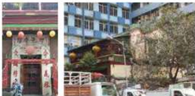
Entrance door of the Sea Ig Temple (R) View of the curved roof of the Sea Ig Temple (Source: Author)
